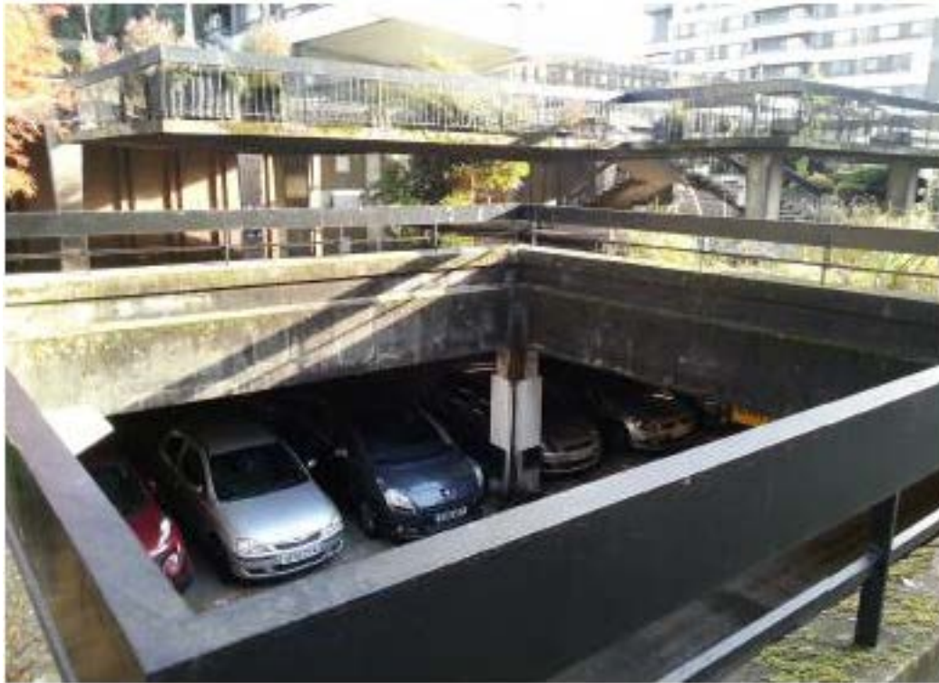
Example of Existing Lightwell
