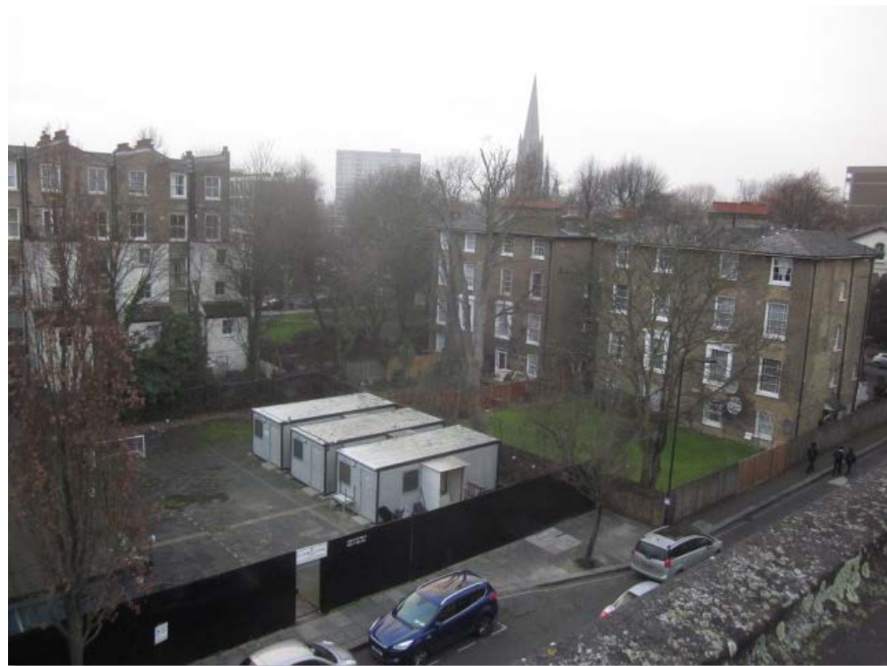
View of Development Site from roof of St George's School
